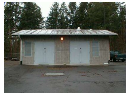
Tacoma Point Well No. 2 Building
