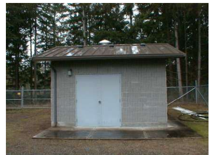
Tacoma Point Well No. 4 Building
